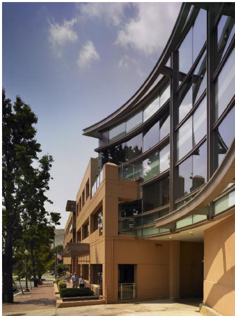
DNC Headquarters Washington, DC
